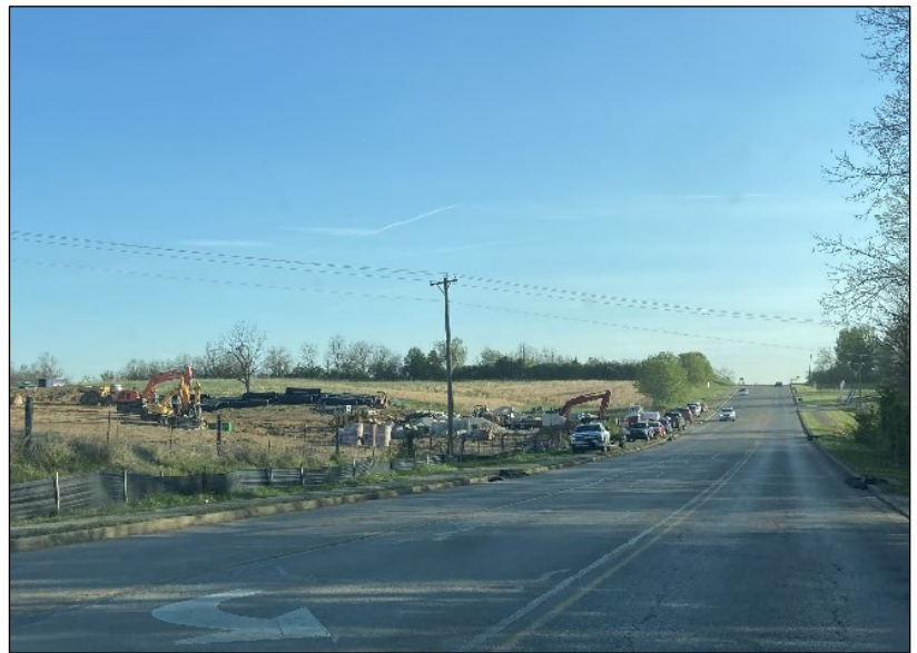
Construction on Goggins Lane
